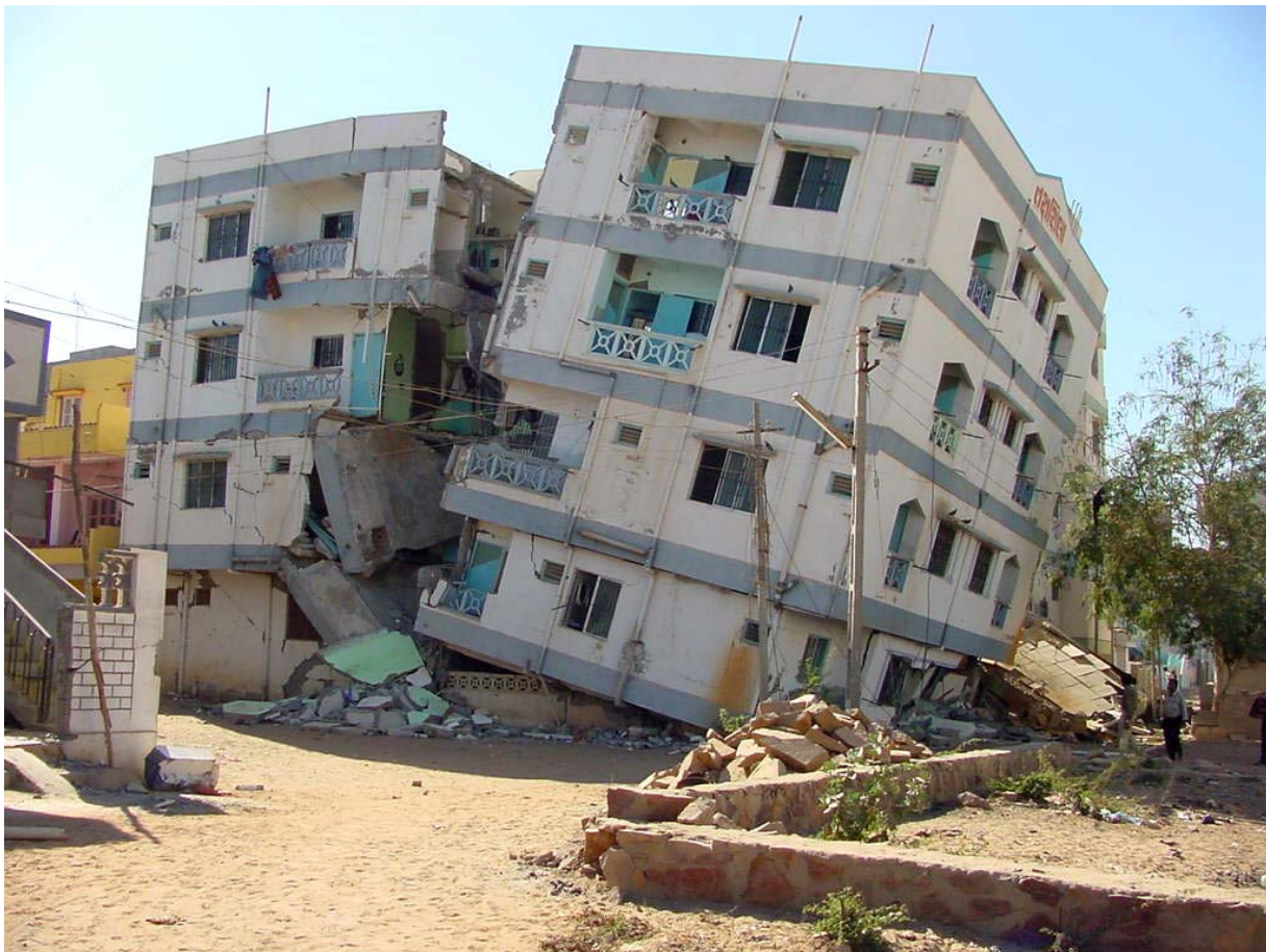
Figure 4.25: Weak storey in a building: collapse of open storey in the five-storey residential building during 2001 Bhuj earthquake (India) in Bhuj town
