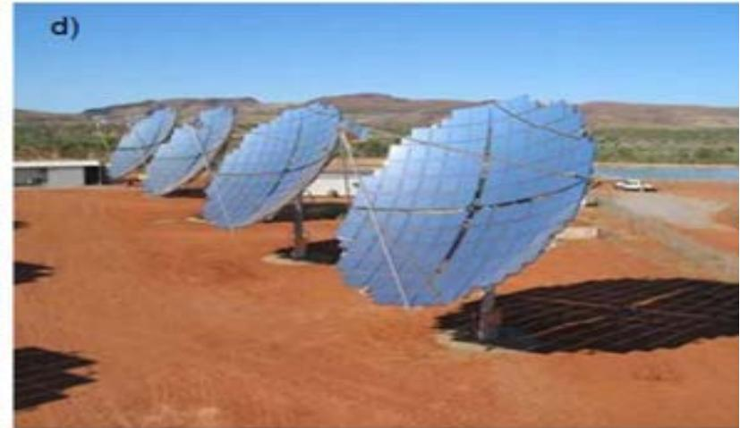
(a) Parabolic Trough, (b) Compact Linear Fresnel, (c) Power Tower and (d) Parabolic Dish.
